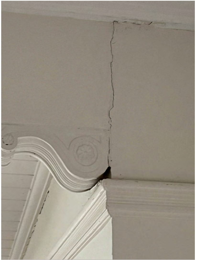
Internal movement and water damage
