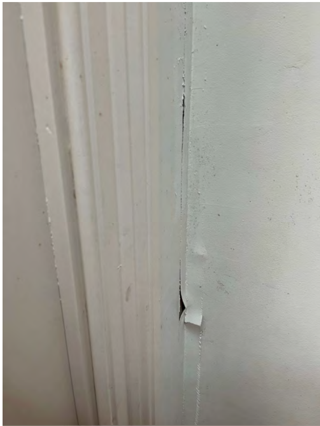
Internal movement and water damage
