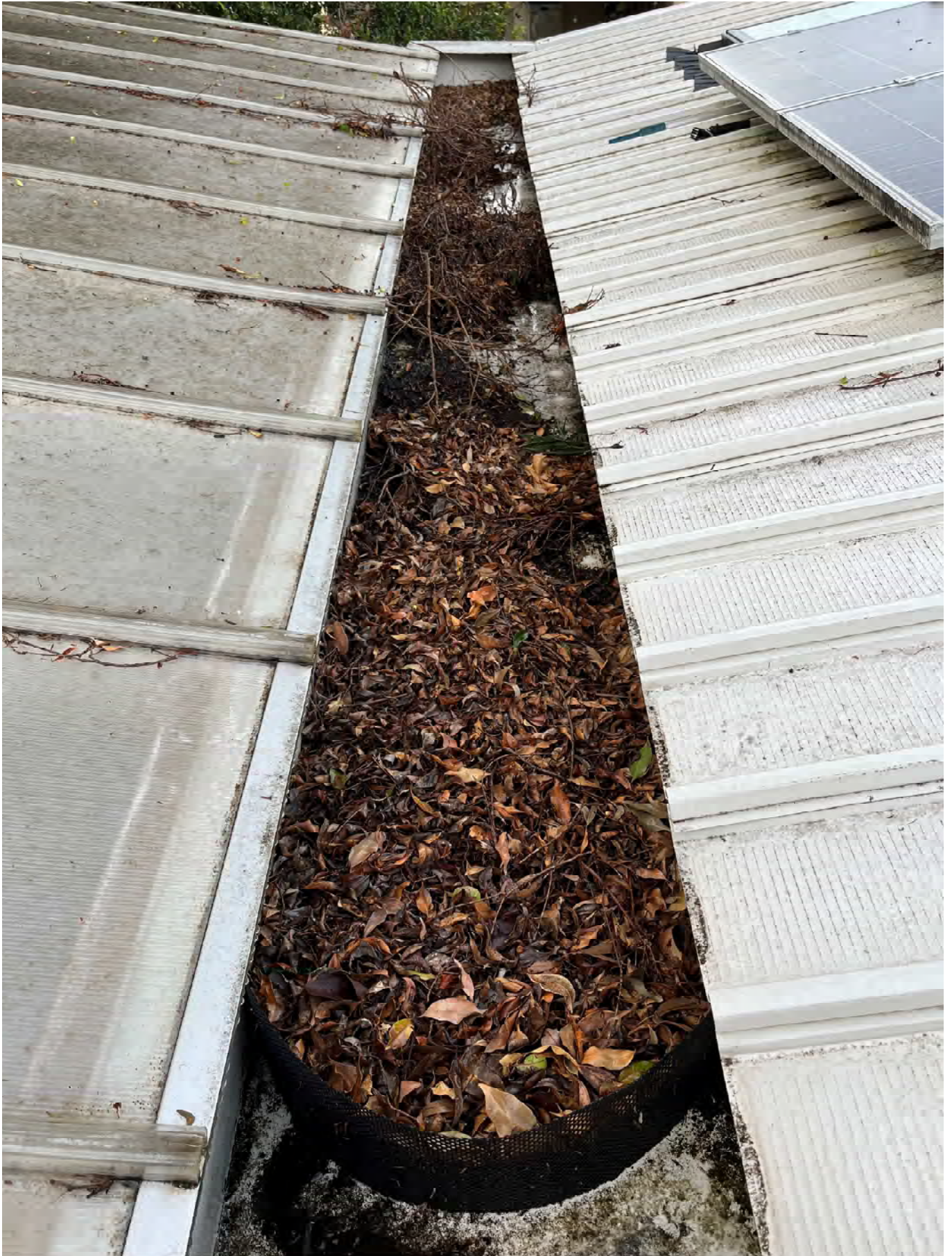
Fallen leaves and branches in new box gutter
